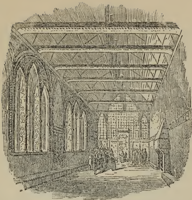
ROOM OF STATE IN THE PALACE
